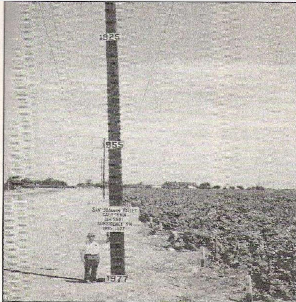
FIGURE 2.3. Land subsidence in the San Joaquin Valley of California. Signs on pole show approximate altitudes of land surface in 1925, 1955, and 1977. Photograph courtesy of the U.S. Geological Survey.
